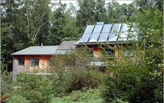
Twin Oaks residence, with solar electricity, solar water heating, passive solar design and super-insulated. Twin Oaks uses about 75% less energy per capita compared to the American average. Twin Oaks is the largest, secular income sharing intentional community in the U.S., and is located in central VA.
