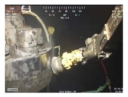
And at this stage, it looks as though they have the bolts loosened - vide the one above the brush, and these below, which appear partly backed out and thus we may already be waiting for the separation tool to come down and remove the old riser. Then the transition spool (under the BOA ROV control) will be moved into place.
