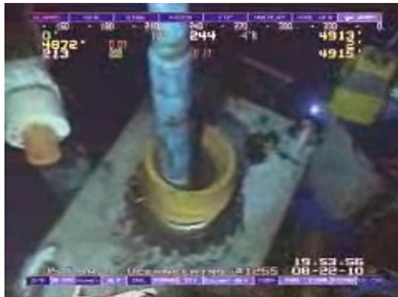
ROV1 guiding pipe in stack
