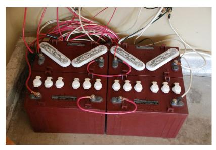
Four golf-cart batteries used in my off-grid home PV system. Each is 12 V, 150 A-h, thus 1.8 kWh of storage apiece.
